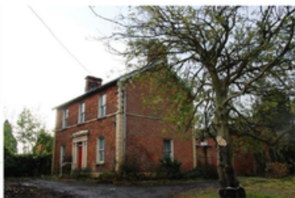
Left: Navigation House, 134 Hillsborough Road, Lisburn © DfC
