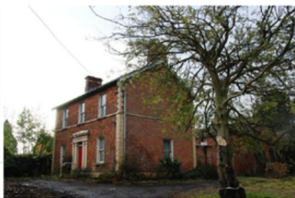
Left: Navigation House, 134 Hillsborough Road, Lisburn © DfC
