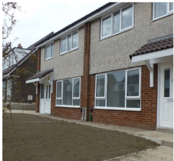
Refurbishment of ex-MOD properties in Lambeg
