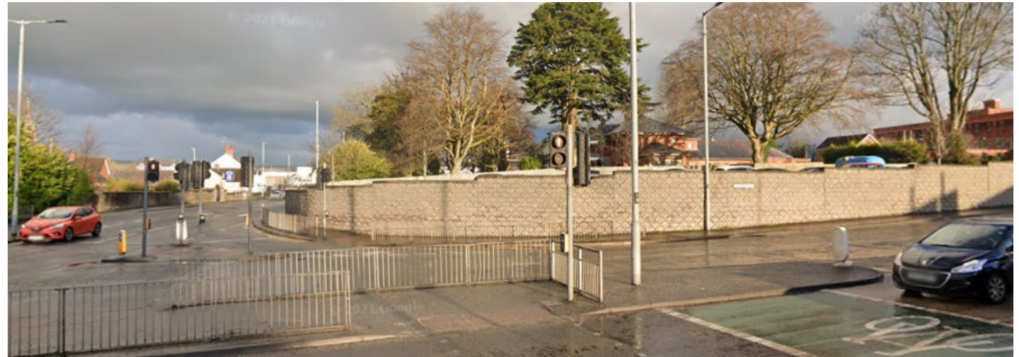
Existing condition: The junction has a large number of barriers, expanses of tarmac and blank wall
